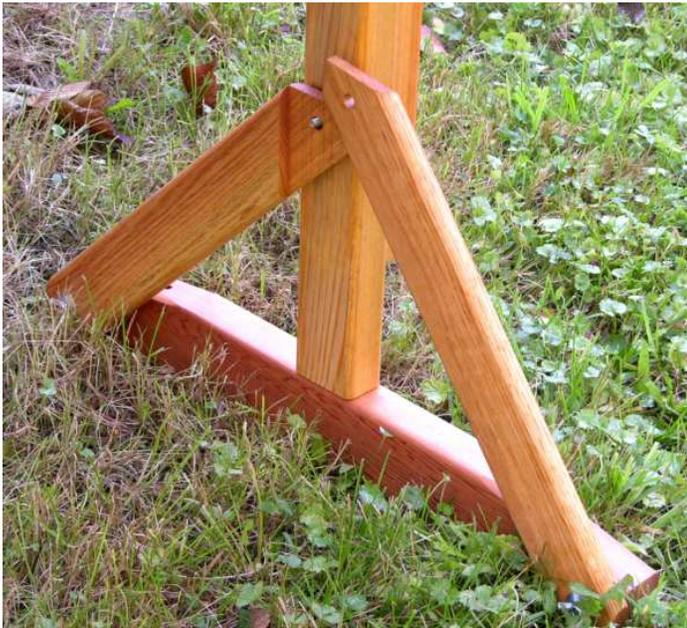
Now is the time to attach the trough. Using the 4" bolts, slide them through the trough and then through the trough support legs. Add a washer and nut to hold the assembly together loosely. You now have the base portion of the feeder together and in good weather it can be used just like this with the roof assembly in storage.
