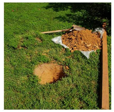
very well. Once done, I went and found a thick flat rock which will now be placed in the bottom of the hole. This is done to give the post a firm strong foundation so it won't sink. Since the rock is 2" thick, I dug out an extra 2" of depth and set the rock in the bottom. Take your post and tap it against the rock several times to seat the rock and make sure the post's bottom sets squarely on top of the rock.
