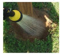
amount of water to dry soil will remove air pockets and help compact the soil. Use very little water to slightly moisten the soil only. Do not create a muddy condition as this will hamper the installation.
