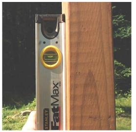
With the post firmly planted but slightly moveable, it is time to level it into its final position. Using a carpenter's level as shown to the left, make sure the post is perfectly level front to back and side to side. As you continue
